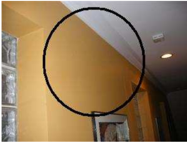
3.2 Picture 1 Basement, North wall
